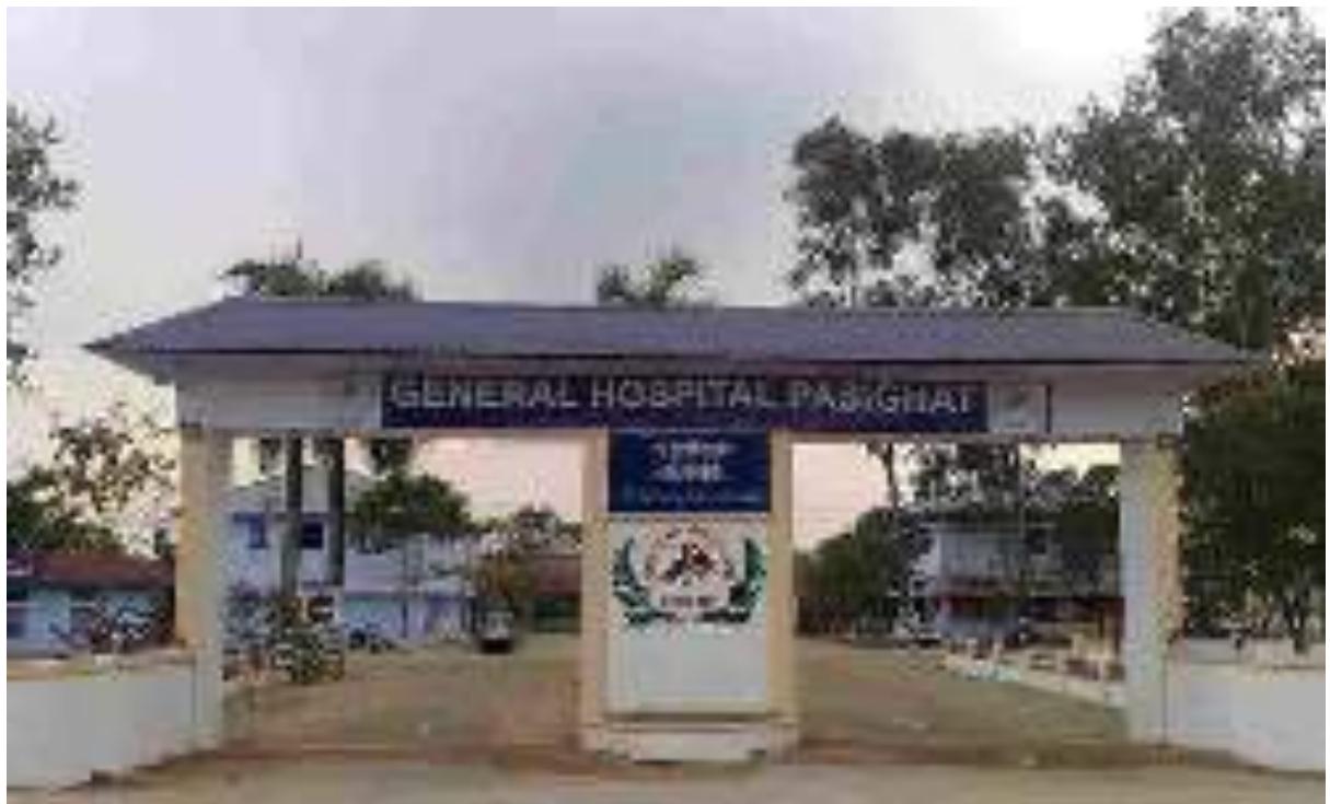
General Hospital, Passighat, East Siang District
